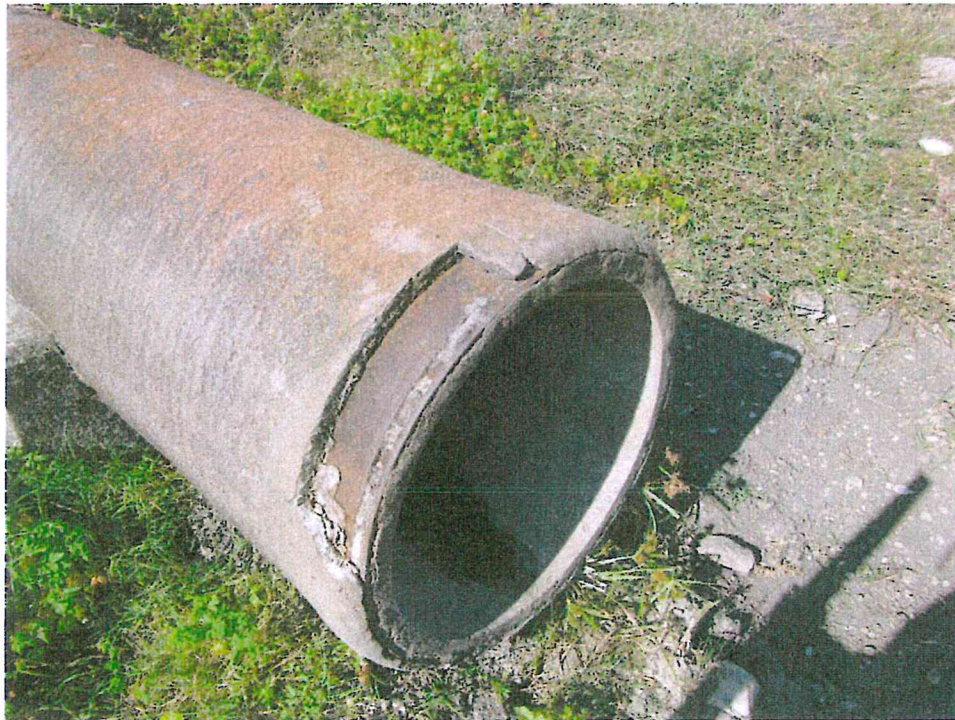
Photograph 12. Principal Spillway discharge outlet with spalling.
