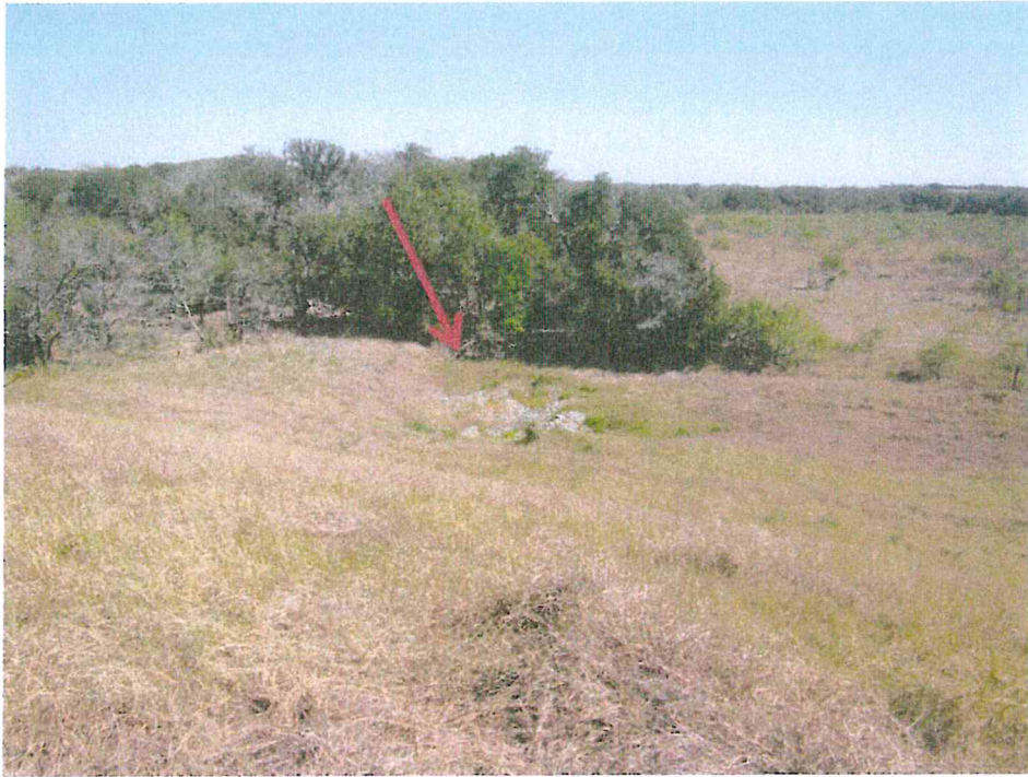
Photograph 15. Discharge channel. Note trees in channel.
