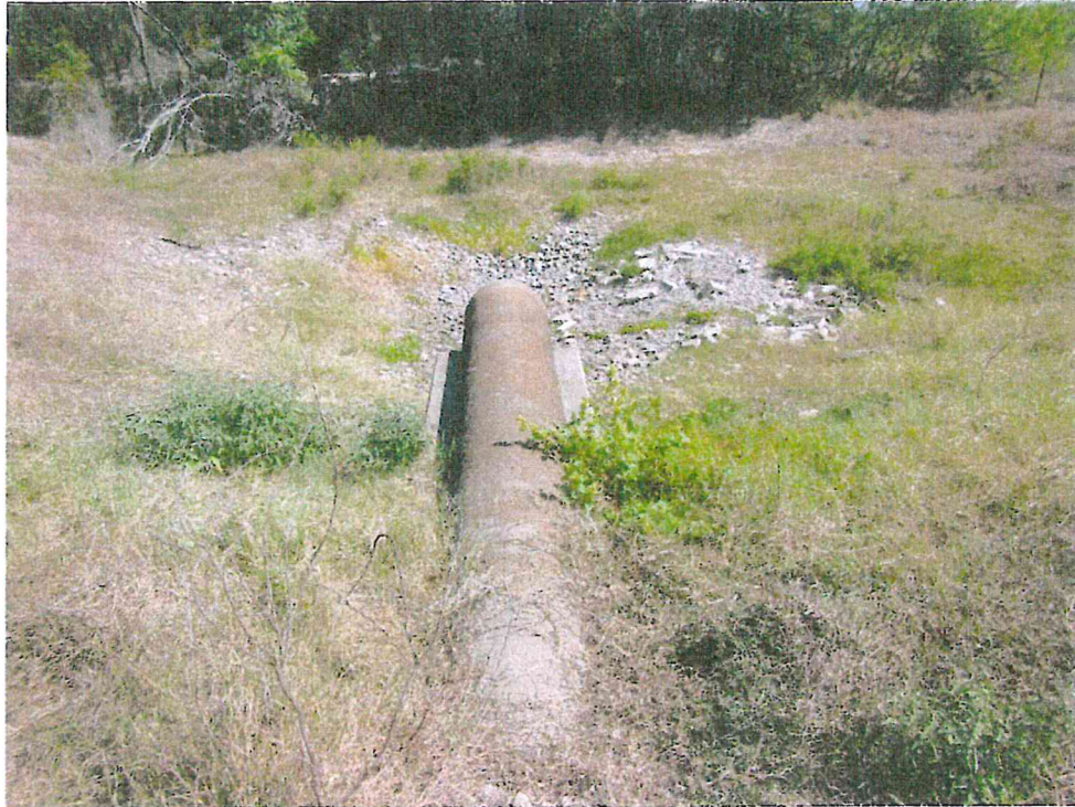
Photograph 13. Principal Spillway discharge outlet and plunge pool.
