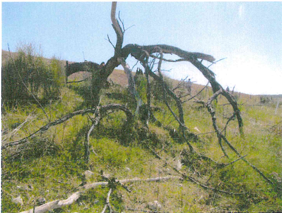
Photograph 4. Upstream slope looking right. Note woody debris.
