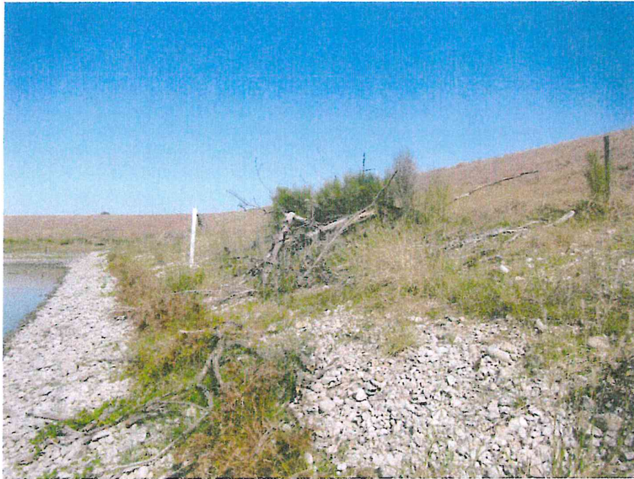
Photograph 5. Upstream slope looking left with dead trees and displaced riprap.
