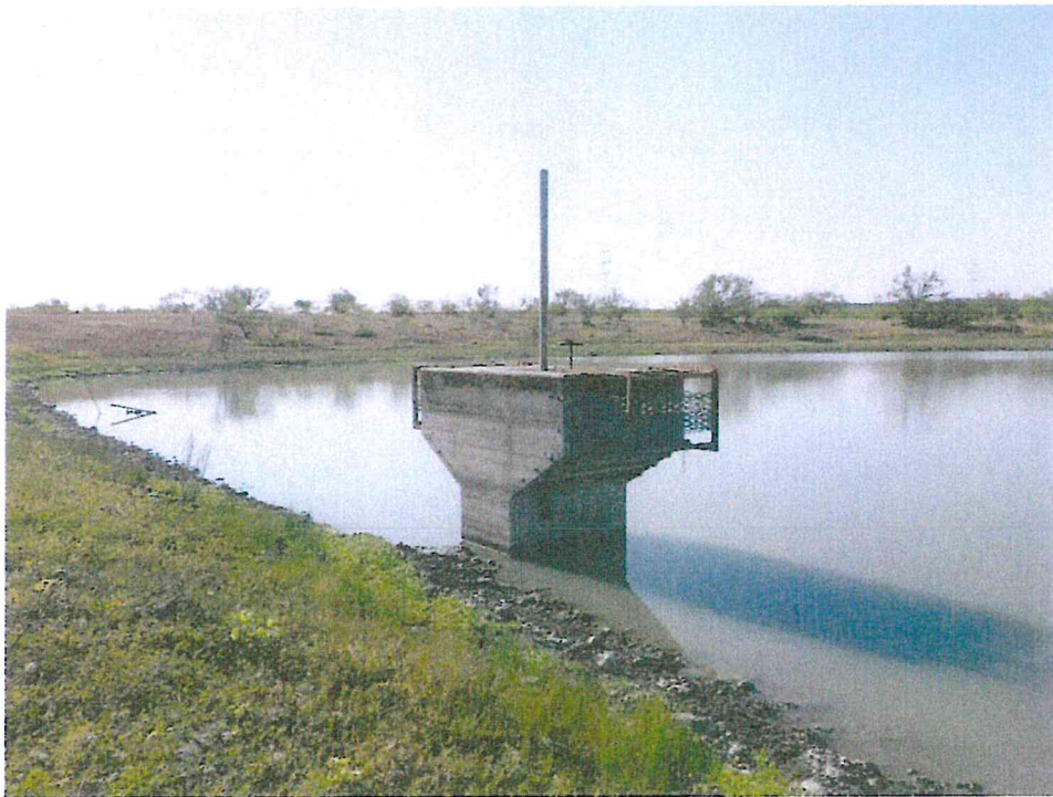
Photograph 10. Principal Spillway inlet.
