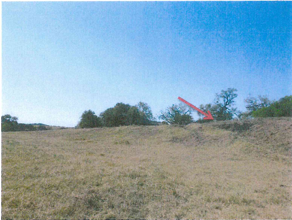
Photograph 11. Emergency spillway northwest crest. Note erosion.
