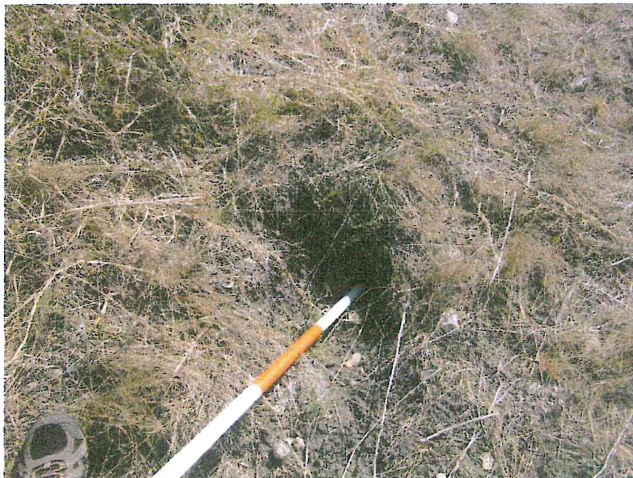
Photograph 6. Upstream slope with burrow.
