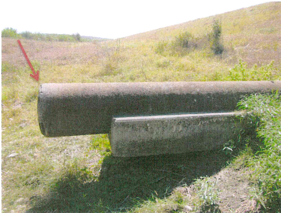
Photograph 14. Principal Spillway discharge outlet with spalling.
