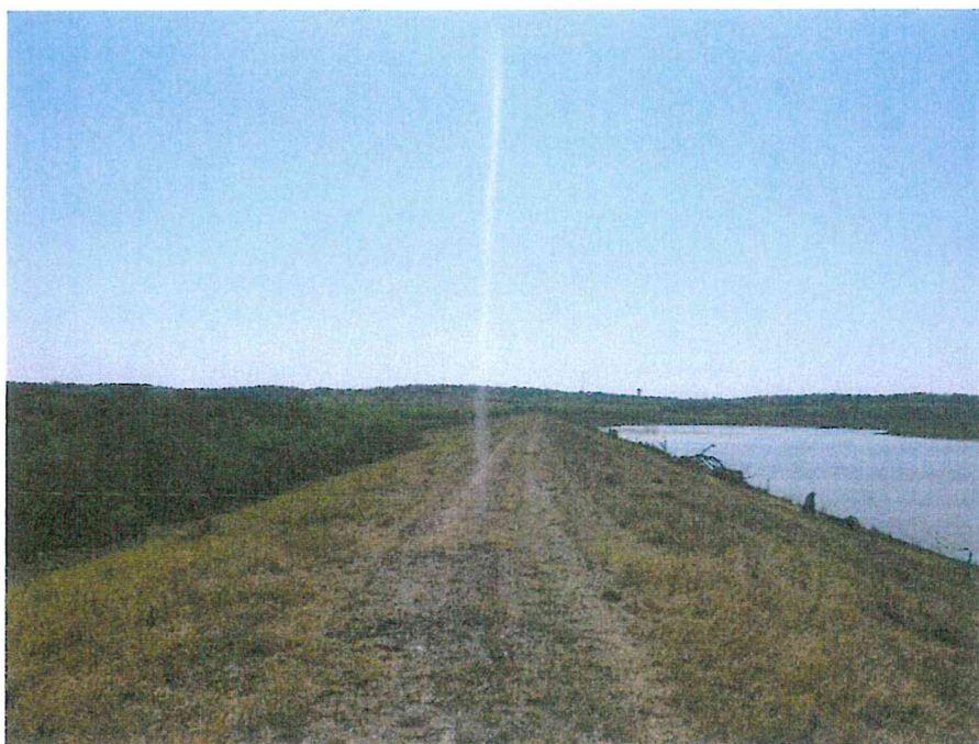
Photograph 1. Crest looking right. Note rutting and bare spots.
