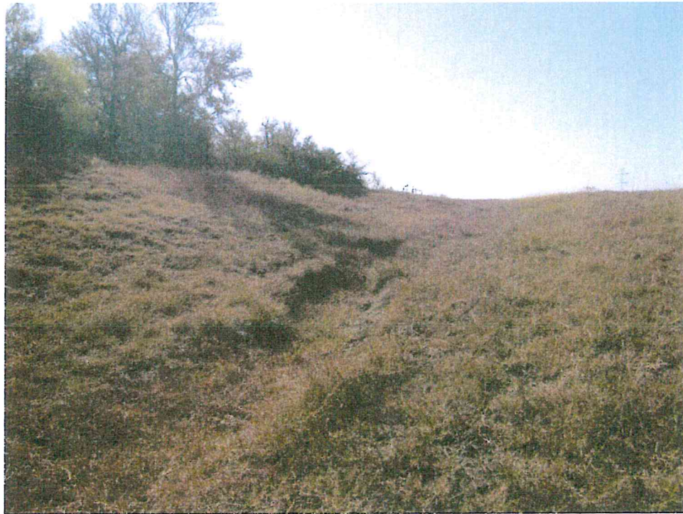
Photograph 16. Emergency spillway outlet. Note erosion.
