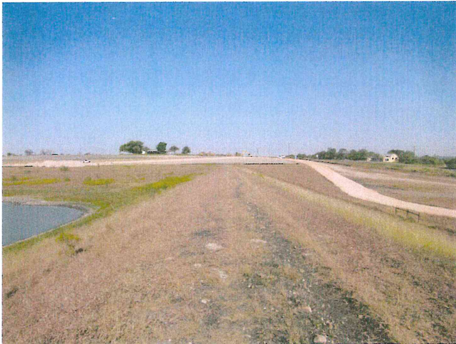
Photograph 2. Crest looking left. Note rutting and bare spots.
