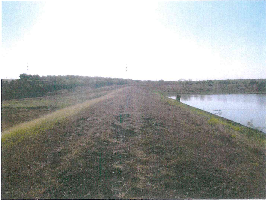
Photograph 1. Crest looking right. Note rutting and bare spots.
