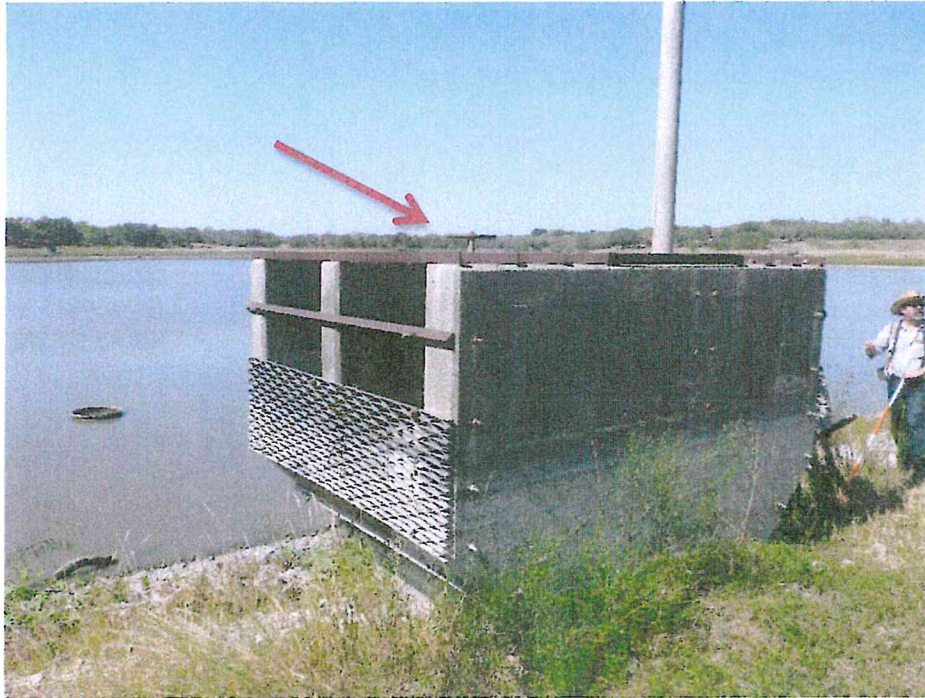
Photograph 9. Principal Spillway inlet and Low Flow valve.
