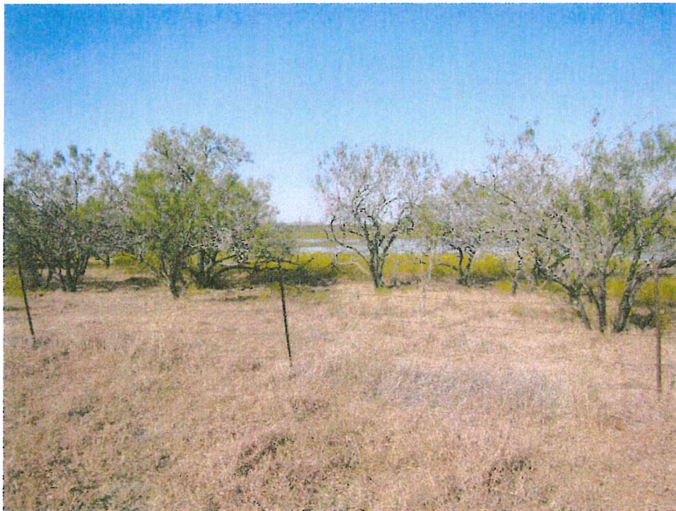
Photograph 14. Emergency spillway inlet. Note trees and fence at inlet.
