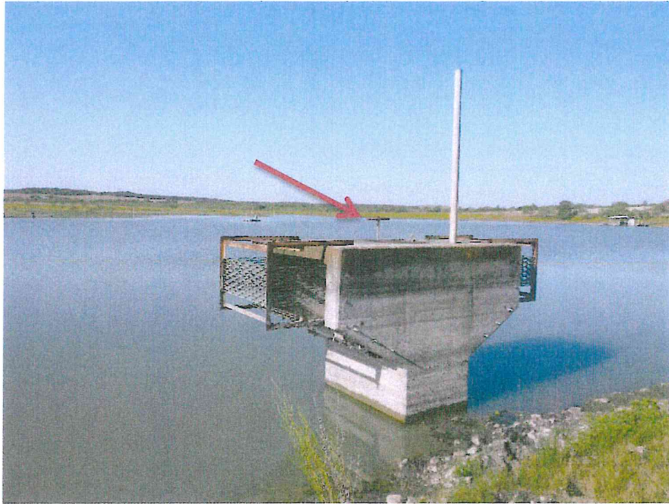
Photograph 11. Principal Spillway inlet and Low Flow valve.
