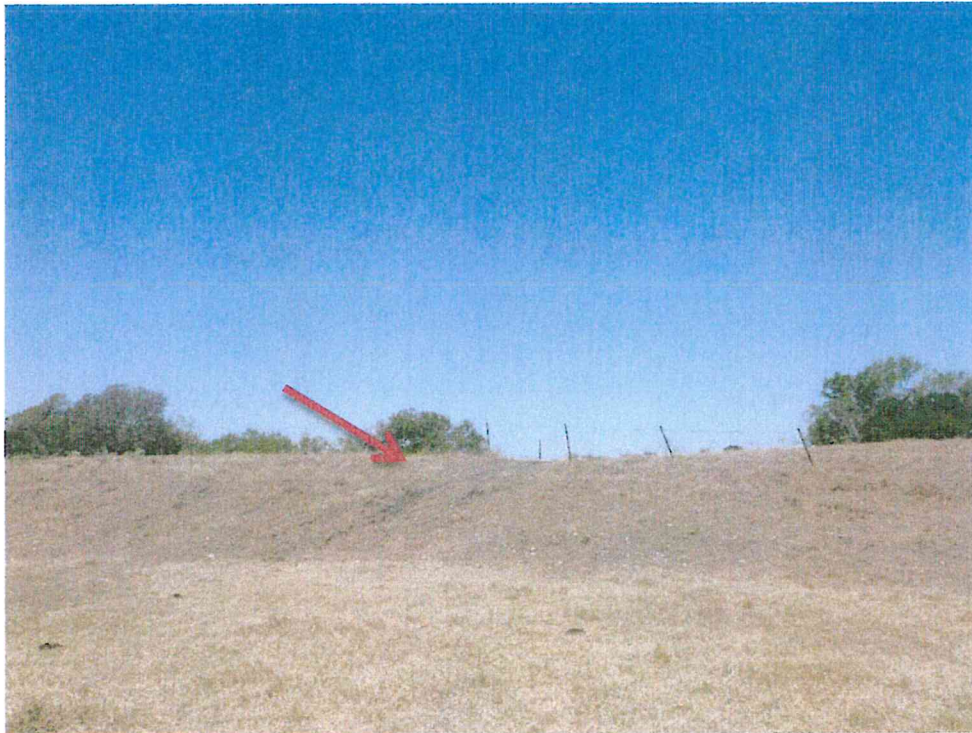
Photograph 12. Emergency spillway northwest crest. Note erosion and damaged fence.
